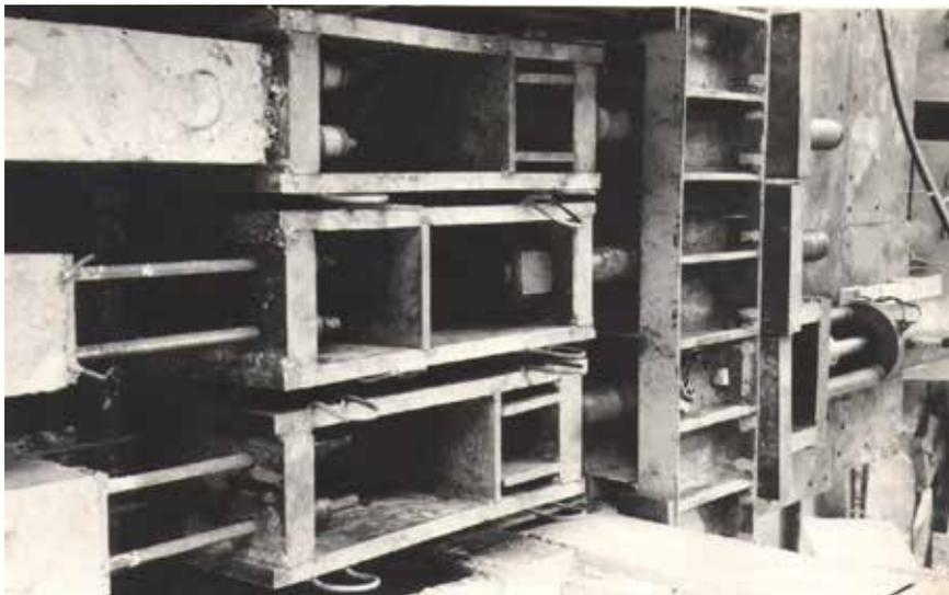
**Fig. 2. Tensioning device for longitudinal steel reinforcement located on the stand in the manufacture of prestressed reinforced concrete beams**
